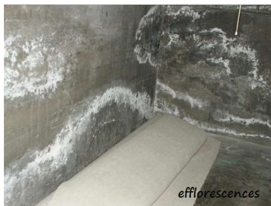
Figure 2: Efflorescence.
